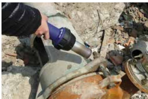
Loosening of screws
